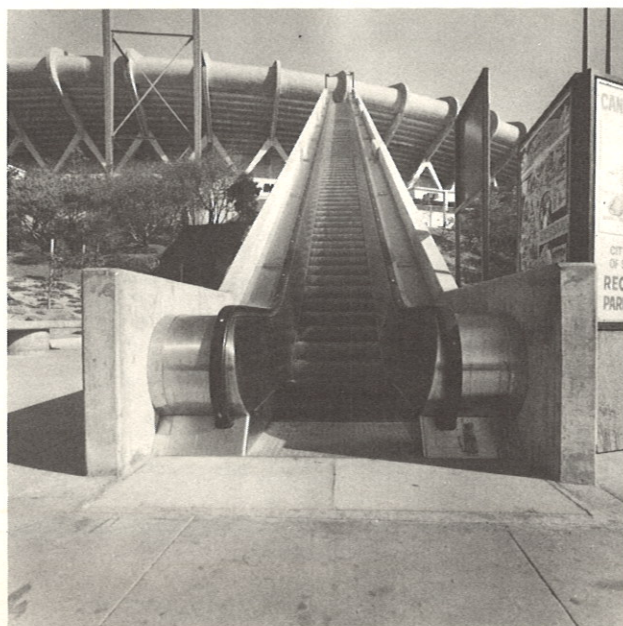
Candlestick Park, San Francisco, California. 6 48" Montgomery escalators, 1 Montgomery traction freight elevator and 2 Montgomery traction passenger elevators.
