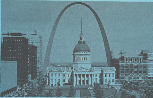
Spectacular Stainless Steel Arch of the Jefferson National Expansion Memorial—St. Louis, Missouri—is the tallest monument in the world. Each triangular leg contains a Montgomery Elevator. Due to the 78 degree angle of the legs, a unique feature, while rising (or descending) the 386 feet of travel, each elevator moves 82 feet horizontally.
