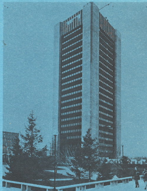
Carleton University — Arts Tower, Ottawa, Ontario. Four Montgomery Gearless Passenger Elevators with speeds of 500 F.P.M. serving 22 floors.
